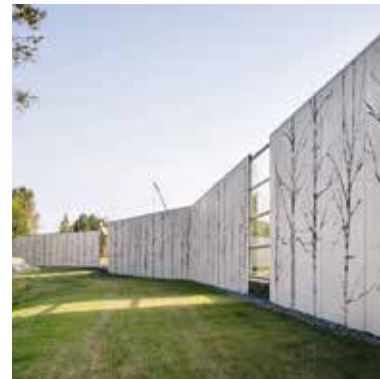
Sound barriers and retaining walls
